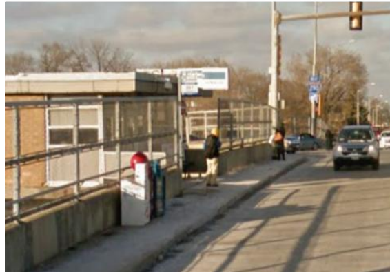
Figure S-6. Existing CTA Access, I-290 at Harlem Avenue
