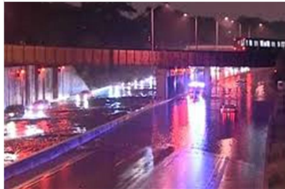
Figure S-7. I-290 Flooding East of DesPlaines Avenue
